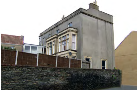
The rear, with added bays and western wing
